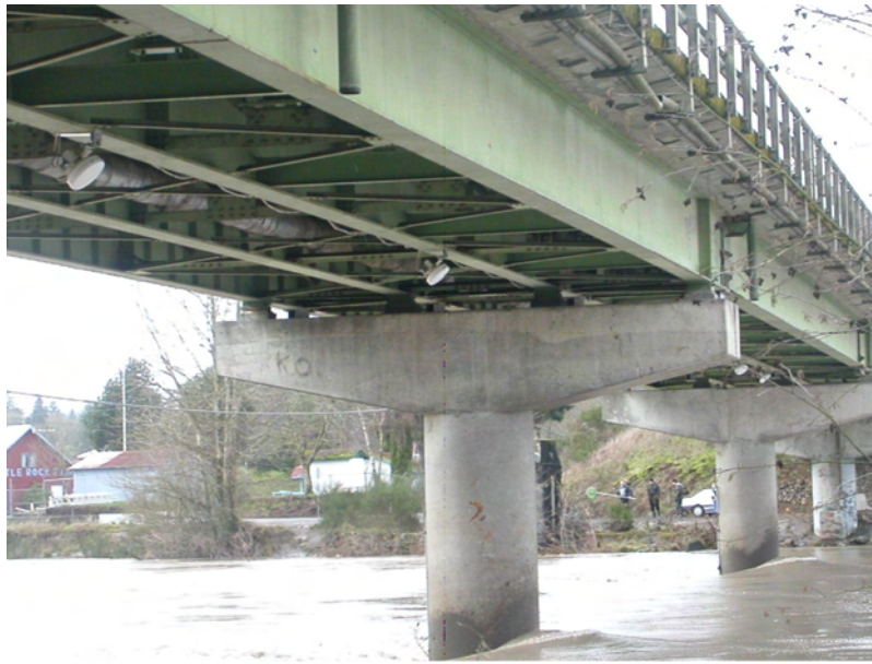
Figure 7. View under Cowlitz River bridge with four of eight RiverScat antennas visible and pointing upstream.
